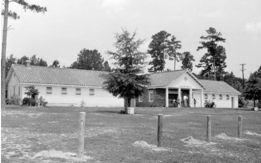
Figure C.7. Bathhouse, June 1947 . The bathhouse's terracotta roof was a design element original to the Civilian Conservation Corps' construction of the park's facilities in the 1930s. Courtesy, Open Parks Network.
