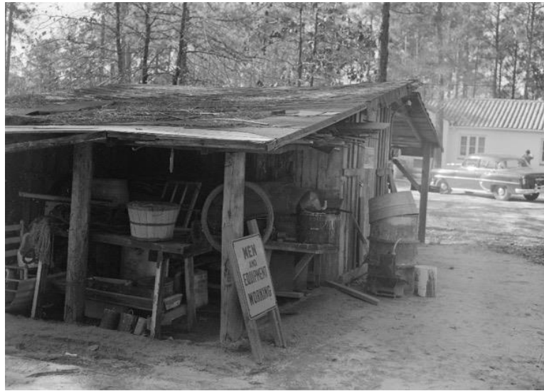
Figure C.5. Old Abandoned Workshop, January 1955. This workshop no longer met the park’s maintenance needs. Today, it no longer exists. Courtesy, Open Parks Network.
