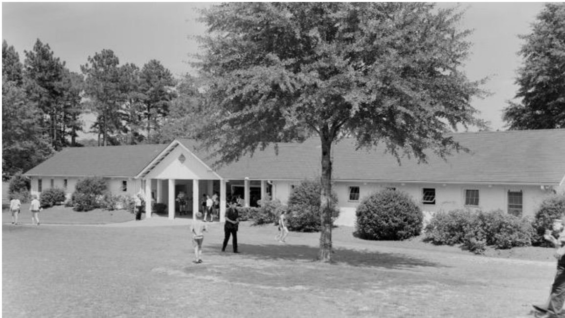
Figure C.8. Bathhouse, Summer 1962 . The replacement of the bathhouse's original roof in 1953 marked a significant change in the appearance of the park's designed landscape. Courtesy, Open Parks Network.
